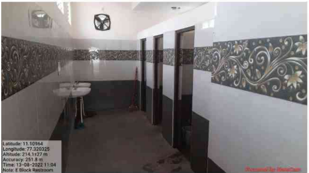
RESTROOM IN E BLOCK
