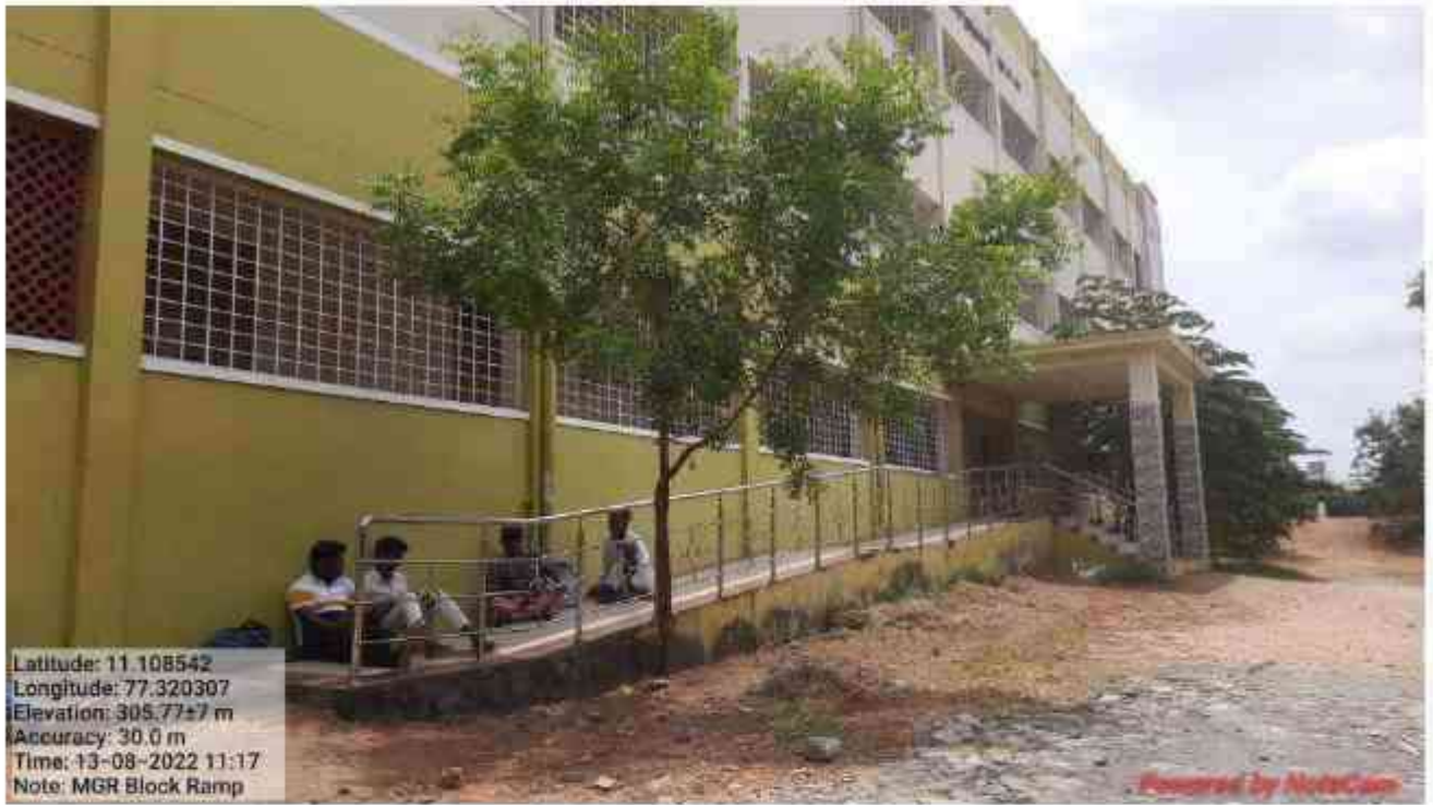
RAMP IN MGR BLOCK
