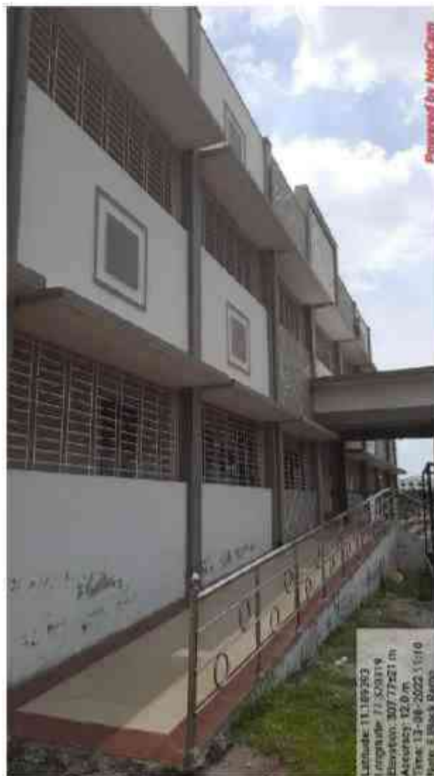
RAMP IN E BLOCK
