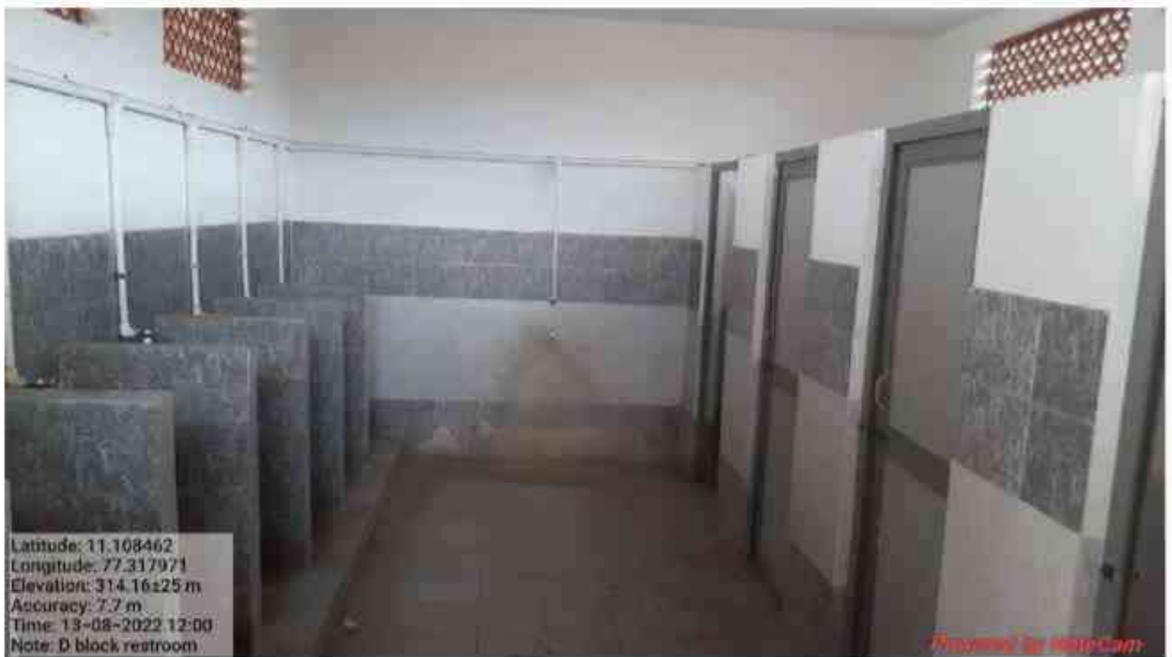
RESTROOM IN D BLOCK.
