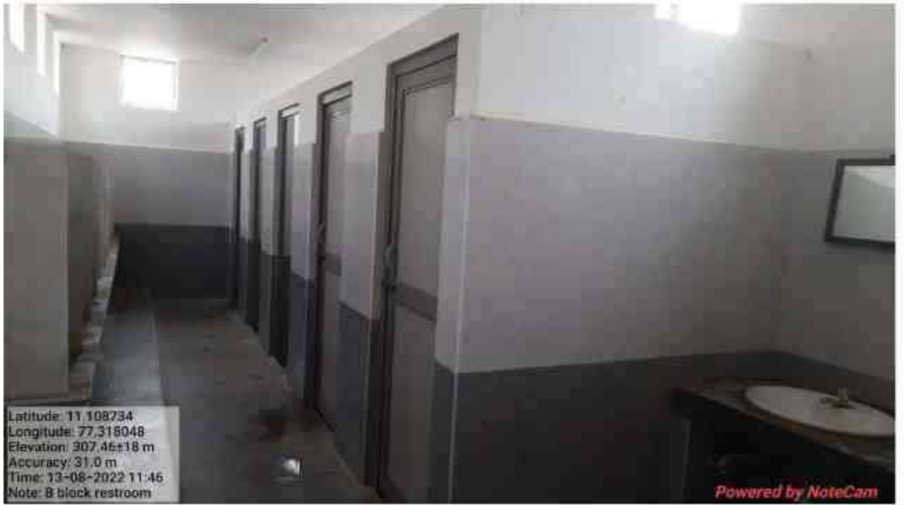
RESTROOM IN B BLOCK
